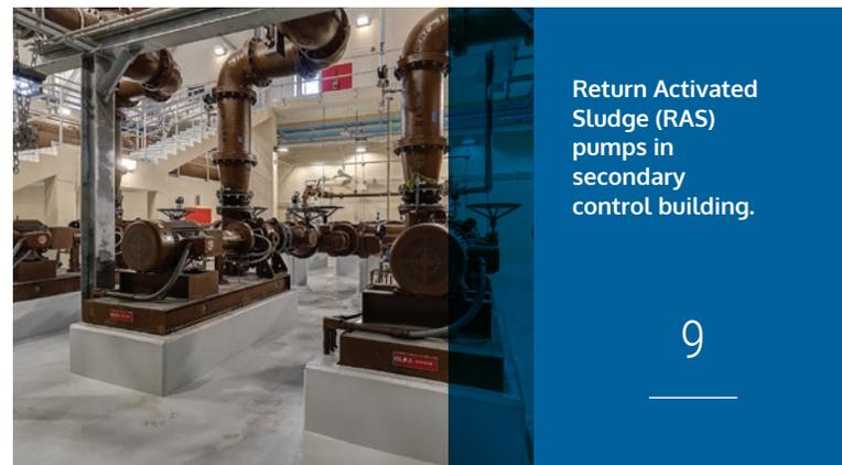
Return Activated Sludge (RAS) pumps in secondary control building.
