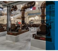
Return Activated Sludge (RAS) pumps in secondary control building.
