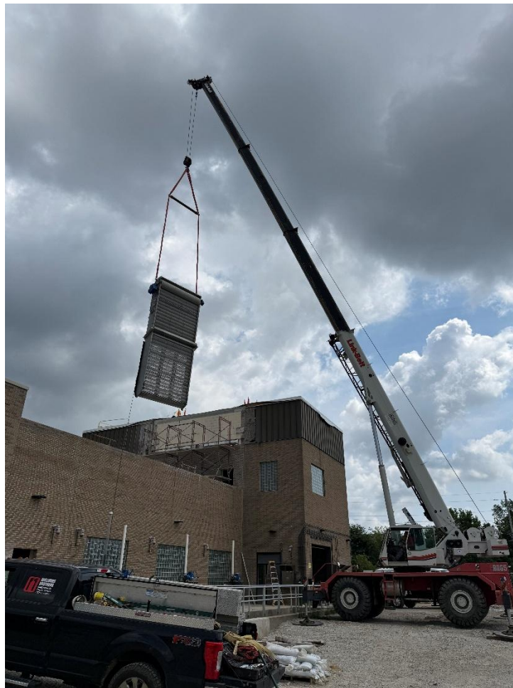
Photo A – Installation of the last screen into the Bar Screen facility
