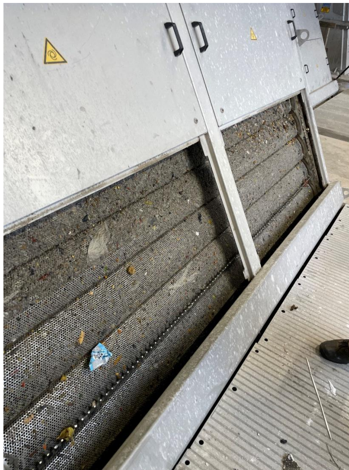
Photo A – Perforated Plate Screen Operation
