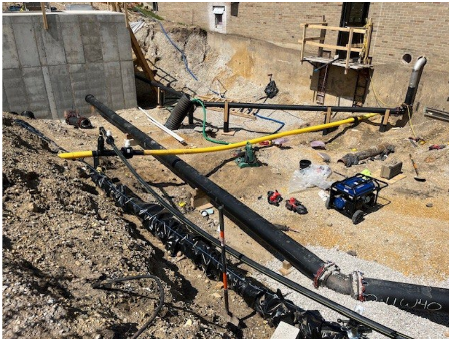
Photo A – New and Existing Underground Piping at Building E
