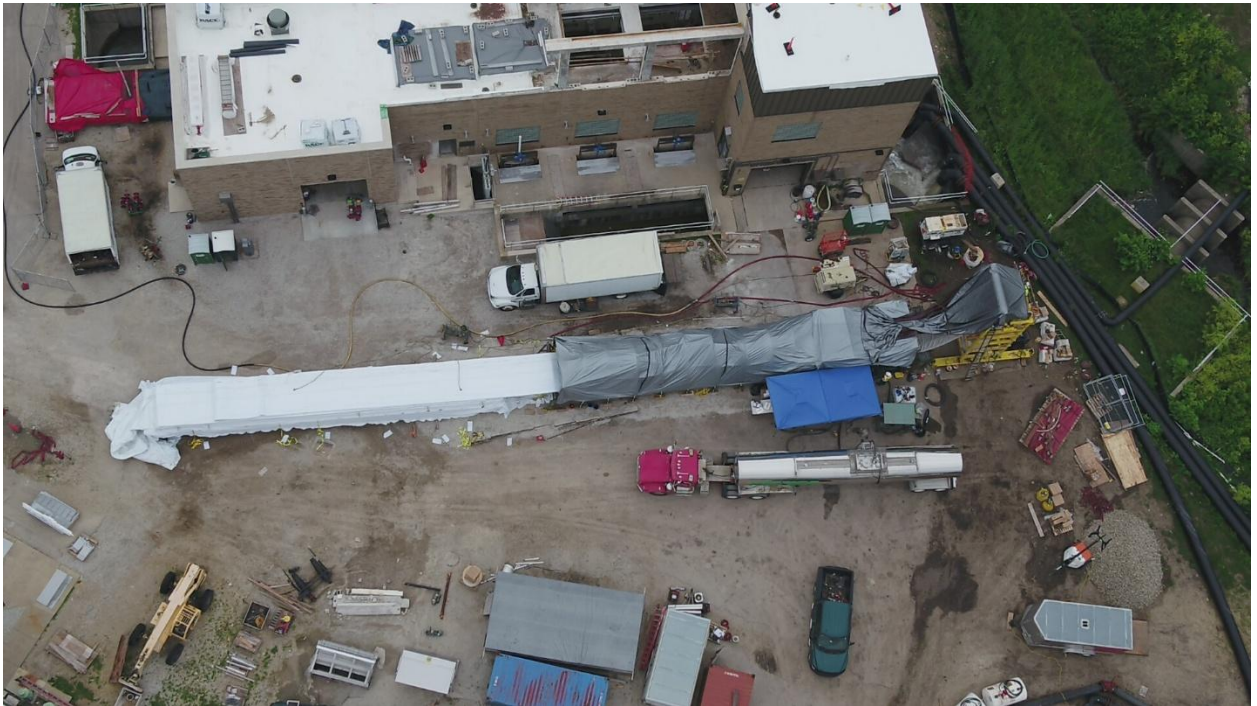
Photo A – OCSI Lining Installation (Aerial View)
